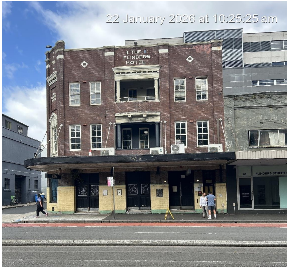
Figure 1: 63-65 Flinders Street, Surry Hills, viewed from the east
